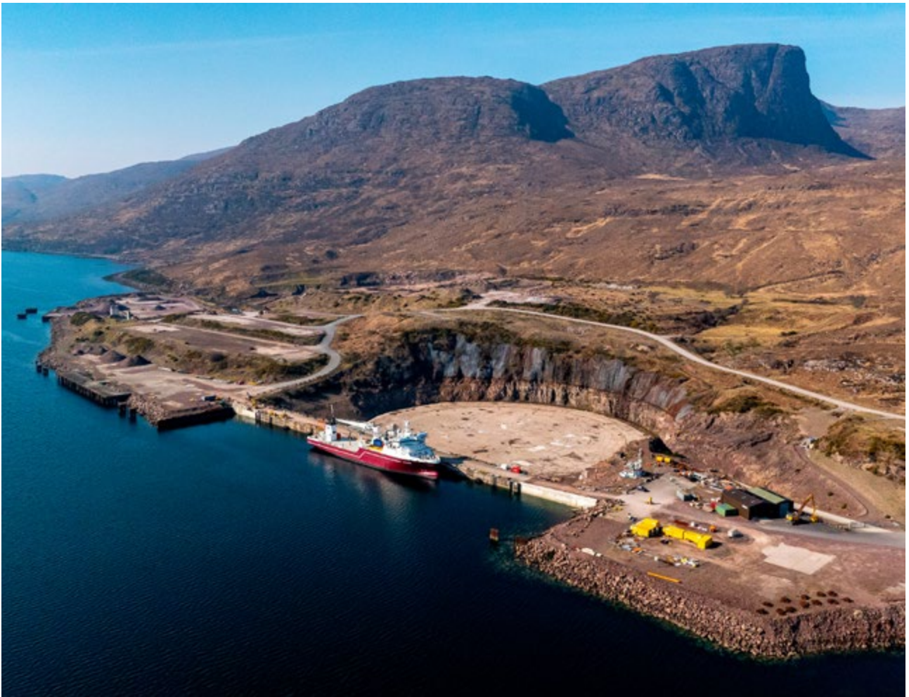
Kishorn Port and Dry Dock, Kishorn
