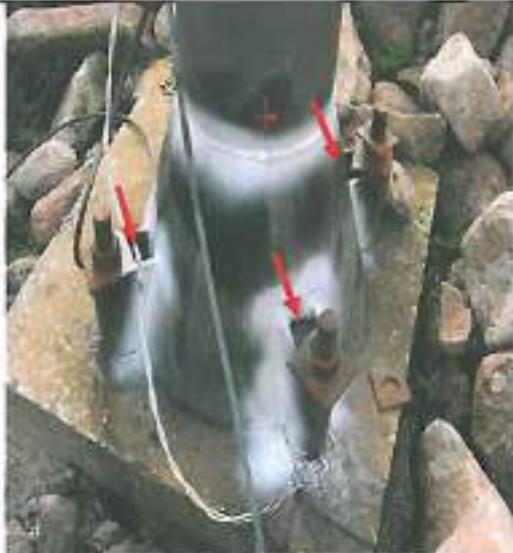
Stand-off Photographic record of Base Plate Cone and Anchor Bolt Housings on tower 2. Restrictions encountered within housings indicated by red arrows.
