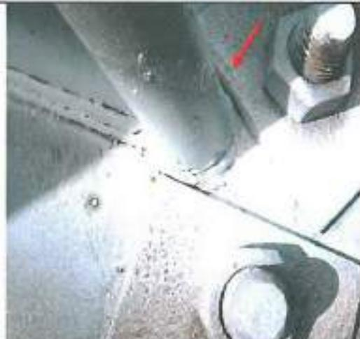
Further Photographic record showing Anchor Bolts and Washers restricting inspection of Weld Cap and HAZ on Tower 6.
