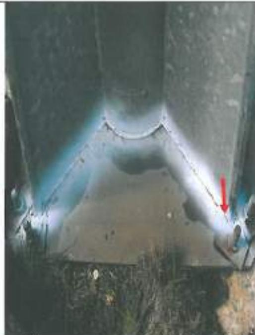
Photographic record showing Deck Plate and Stiffener welds with Anchor bolts on Tower 2.
