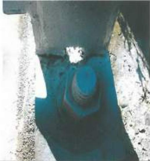
Photographic record showing base plate connection welds from angled lattice work and anchor bolt on T1L (facing down-hill).
