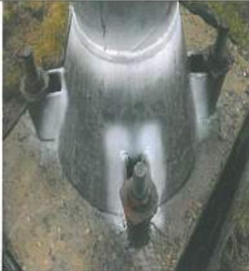
Photographic record of Base Plate Cone and Anchor Bolts and Housings on Tower 2.
