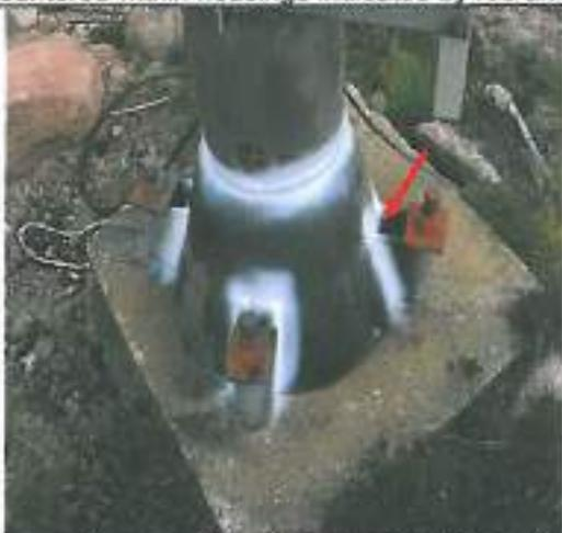
Photographic record showing extent of Magnetic Particle Inspection area at Base Plate Cone to Tower and Housing Welds and Anchor Bolts on Tower 6.
