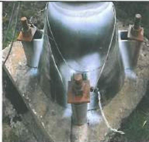
Photographic record showing Anchor Bolts/Washers and Cone to Tower Weld on Tower 9. High tensile wires are termination points for snow fences following the tow up the hill.
