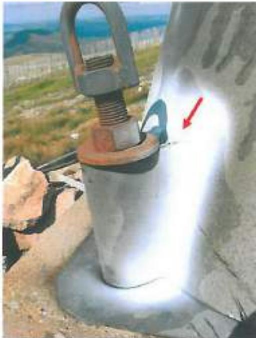
Photographic record of Base Plate and Anchor Bolt Housing on Tower 2. Restrictions were encountered on internal Base Cone Connection from Anchor Bolt Housing.
