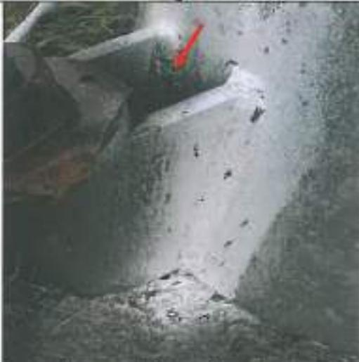
Photographic record of Base Plate Cone and Anchor Bolts and Housing on Tower 15. Arrow indicates restricted access to internal Anchor Bolt Housing.
