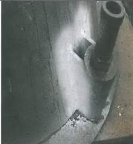
Photographic record of Base Plate and Anchor Bolt Housing on Tower 3. Restrictions encountered on internal Anchor Bolt Housing.
