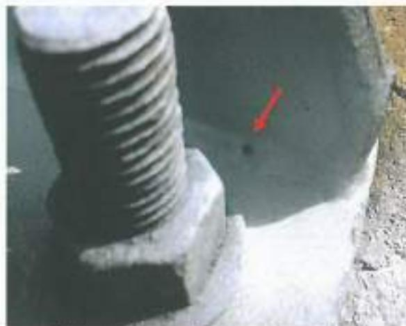
Photographic record showing Porosity on Stiffener Deck Connection weld on Right hand side down-hill Stiffener on Tower E.
