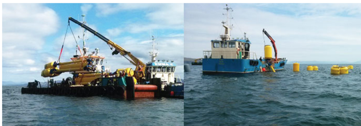
FIGURE 12: ALBATERN ENERGY ARRAY - INSTALLATION
