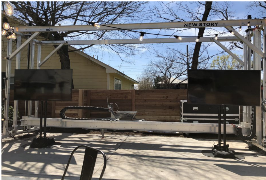
Figure 2.20 Vulcan concrete printer (2018)
