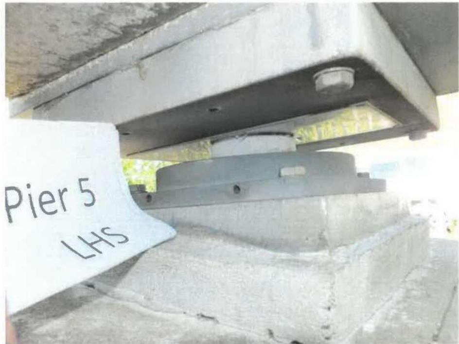
Figure 7 Example of free sliding bearing with tapered bottom plate.
