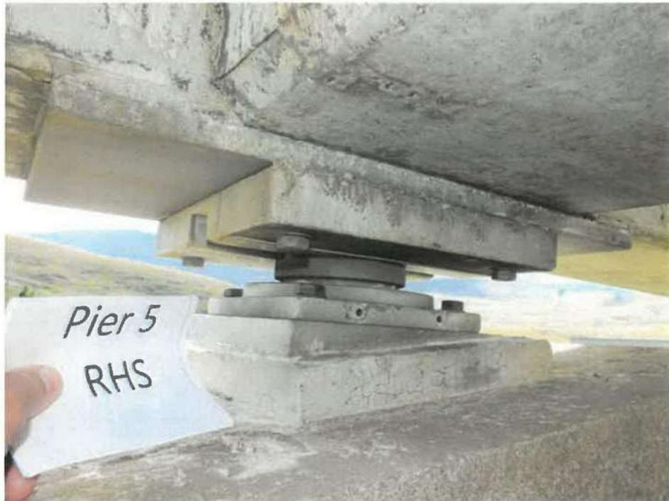
Figure 8 Example of guided bearing with tapered bottom plate
