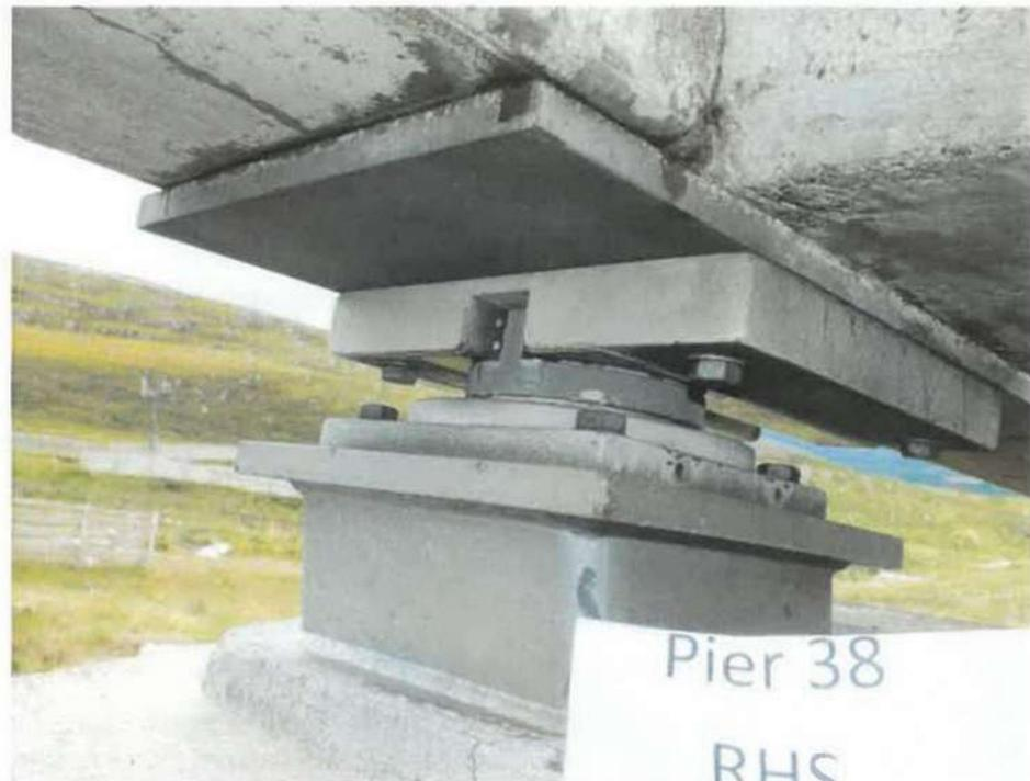
Figure 10 Example of guided bearing with bottom steel shoe
