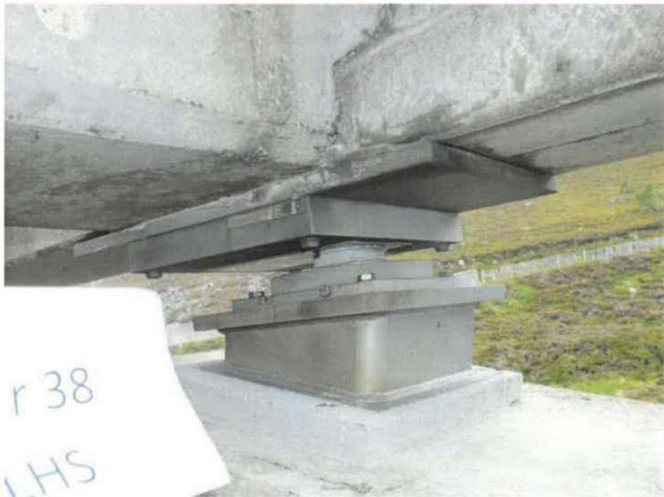
Figure 9 Example of free sliding bearing with bottom steel shoe
