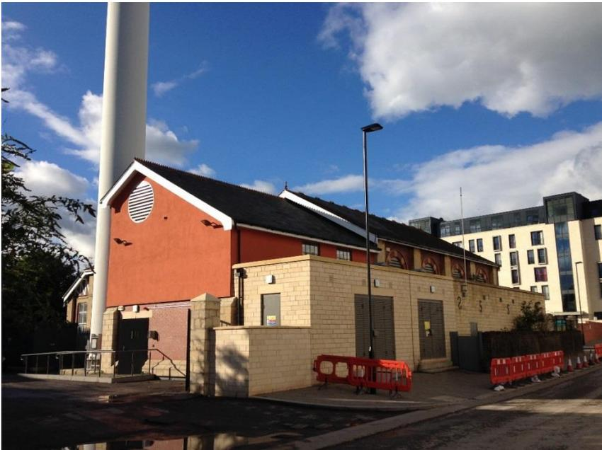
Figure 1: Gas CHP Energy Centre providing heat to approximately 2,000 flats
